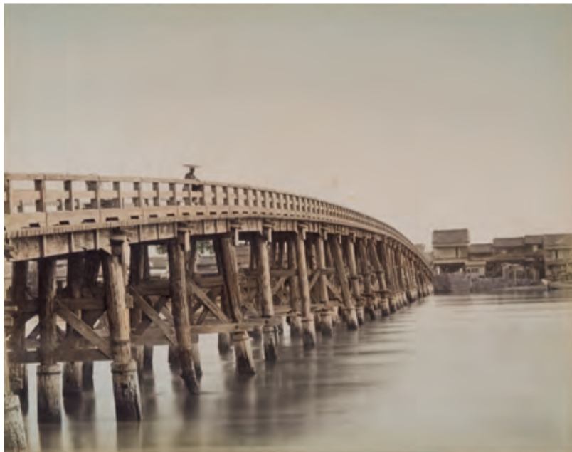
Photograph: Eitaibashi Bridge Early Meiji period
